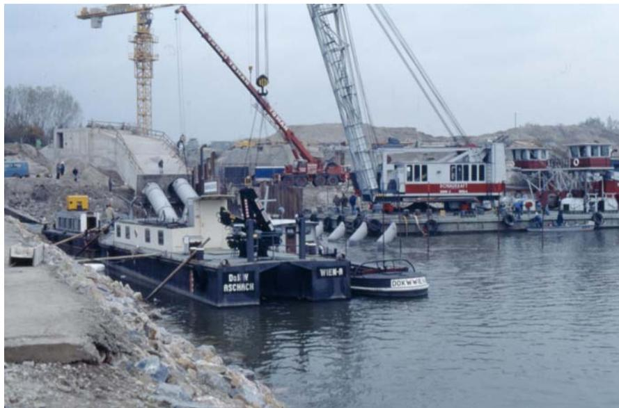
Fig.4: mounting of second feeder pipe
